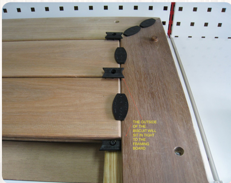
Butt Joiners - for mitred corners, picture frame joints, Butt Joints - as used by cabinet makers this makes it stronger
